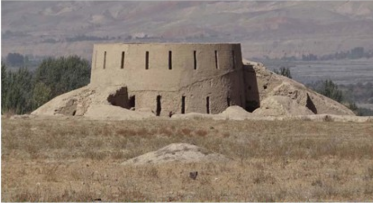
SANJAR SHAH CITADEL, POST-RESTORATION (2014)
